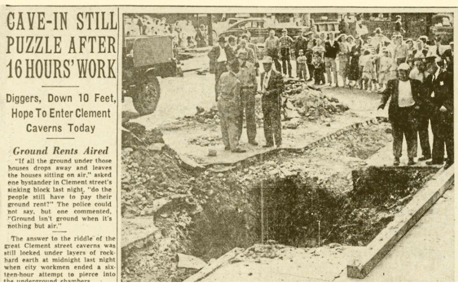
In 1951, City workers dug through the pavement on the 600 block of E. Clement Street to discover long-forgotten caverns. Baltimore Sun photo (June 12, 1951).
