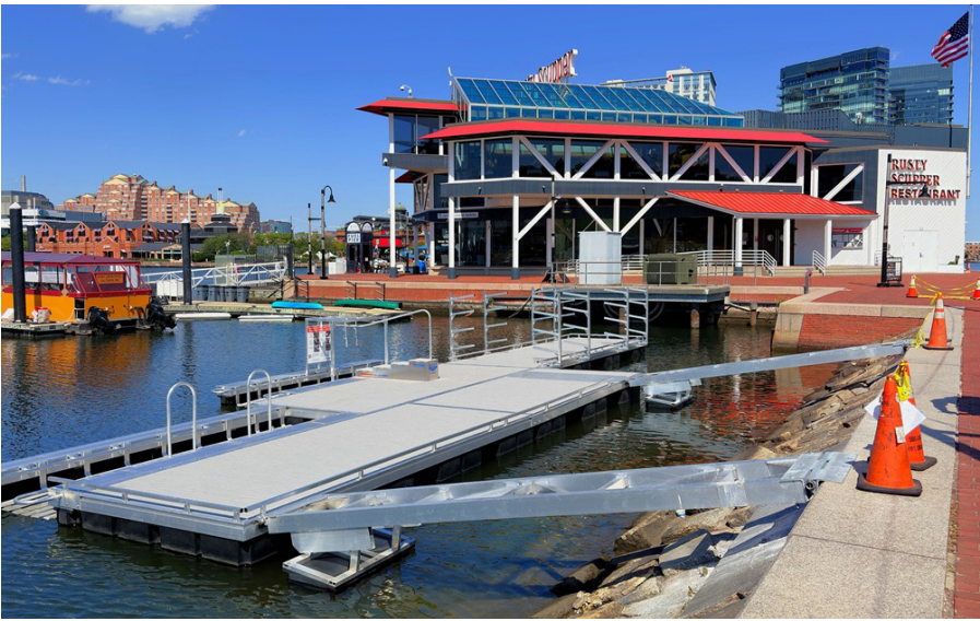
The newly installed public kayak launch along the Inner Harbor’s “Baltimore Blueway” will feature self-service kayak rentals. Photo by Mary Braman.
