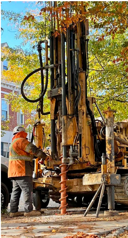
Soil borings up to 40 feet deep were drilled through the sidewalk on the 600 block of E. Clement Street in November. Photo by Steve Cole.
