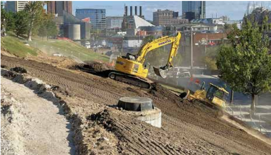
Work to reshape and stabilize a section of the side of Federal Hill Park overlooking Covington Street started in August to address persistent erosion issues.
