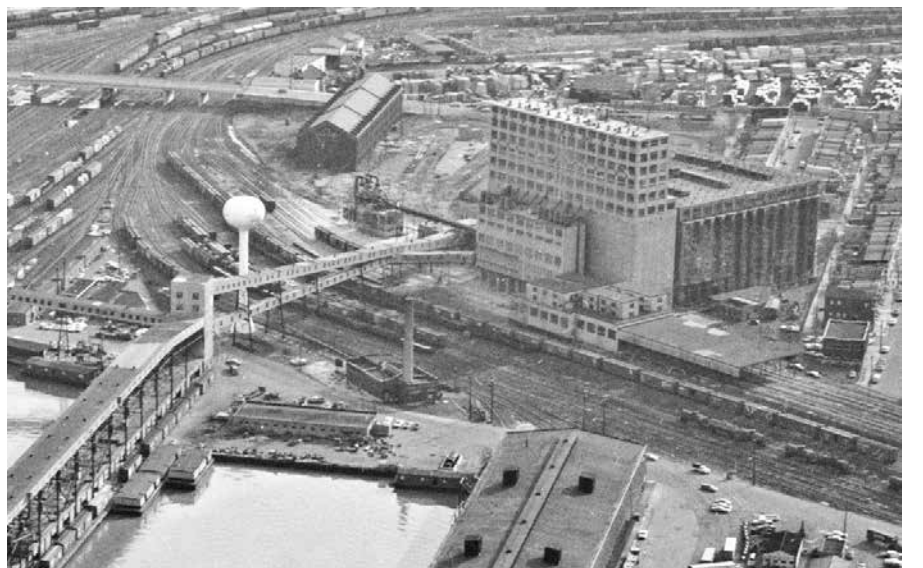
The massive grain elevators built in Locust Point by the B&O Railroad 100 years ago replaced wood-framed elevators that were destroyed by fire. The structure was converted into the Silo Point condominiums. Photo below: Courtesy Baltimore Museum of Industry Archives. Photo above: Baltimore Sun, Sept. 9, 1924.
