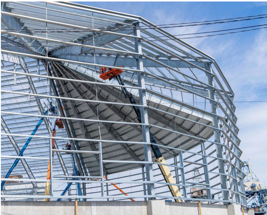
STEEL WAS RISING this summer on the new raw sugar warehouse at the Domino refinery along Key Highway East. By late July, the roof and walls were being added to the structure, which replaces the warehouse that burned in April 2021. The new warehouse will be able to hold 100 million pounds of sugar and is expected to begin operations in early 2025. Photo by Mary Braman.
