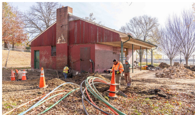
The extensive Riverside Park renovations begun in September 2022 involved constructing a drainage system across the playing fields, covering the fields with new sod, creating new basketball and pickleball courts, and upgrading utilities to the red field house, which will now have bathrooms. Photos by Mary Braman.
