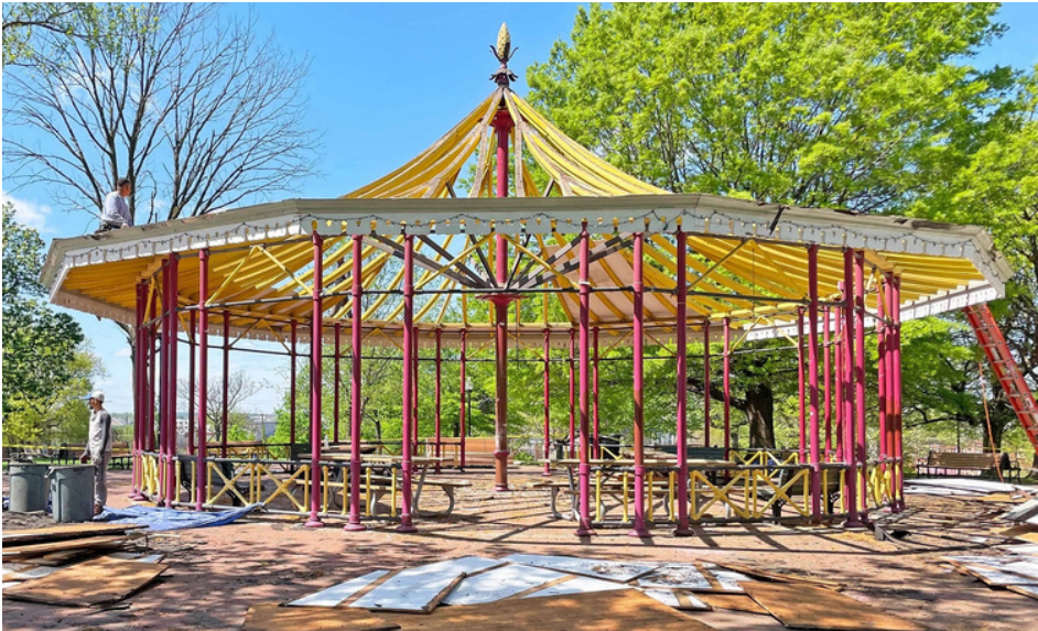
THE RIVERSIDE PARK GAZEBO received a new roof in mid-April as part of a restoration project funded by the South Baltimore Gateway Partnership. A new coat of paint is coming by the end of June. New cast iron bases for the columns are being fabricated. The entire restoration is expected to be completed by September. The project is managed by Baltimore City Recreation and Parks. Photo by Mary Braman.
